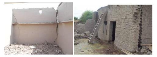
Fig. 5. Damaged houses due to splitting of corners.
