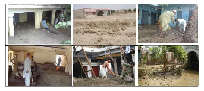
Fig. 8. Damaged houses due to deposition of debris after floods.
