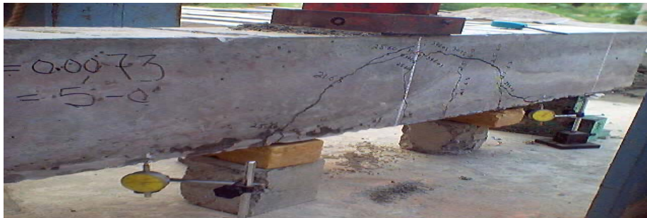
Figure 4. Typical flexural failure mode of the beam at minimum longitudinal steel and no web reinforcement. ( \rho = 0.33\% , a/d = 3.00 , span=152cm)
