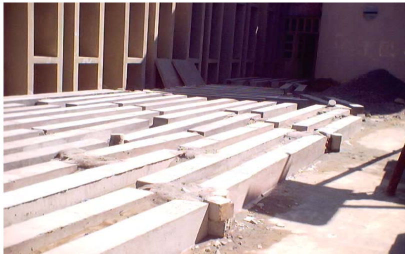
Figure 3. Beams are stacked in the testing yard after casting and curing
