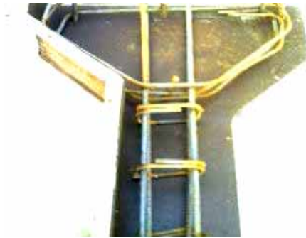
Figure 3. Corbel form work and reinforcement
