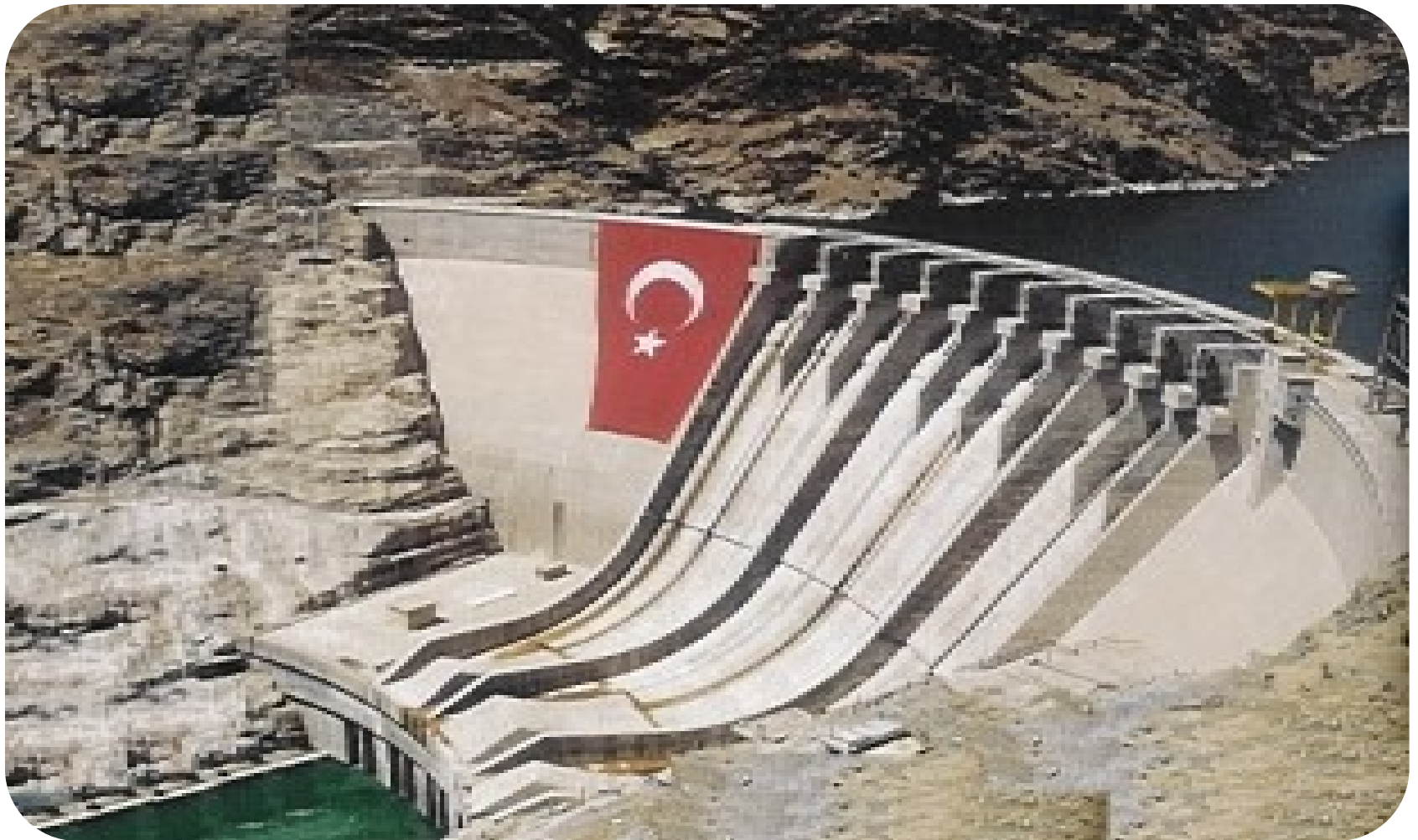
Karakaya Dam – Fırat River; Height= 173 m Reservoir Capacity= 9,5 billion m 3
